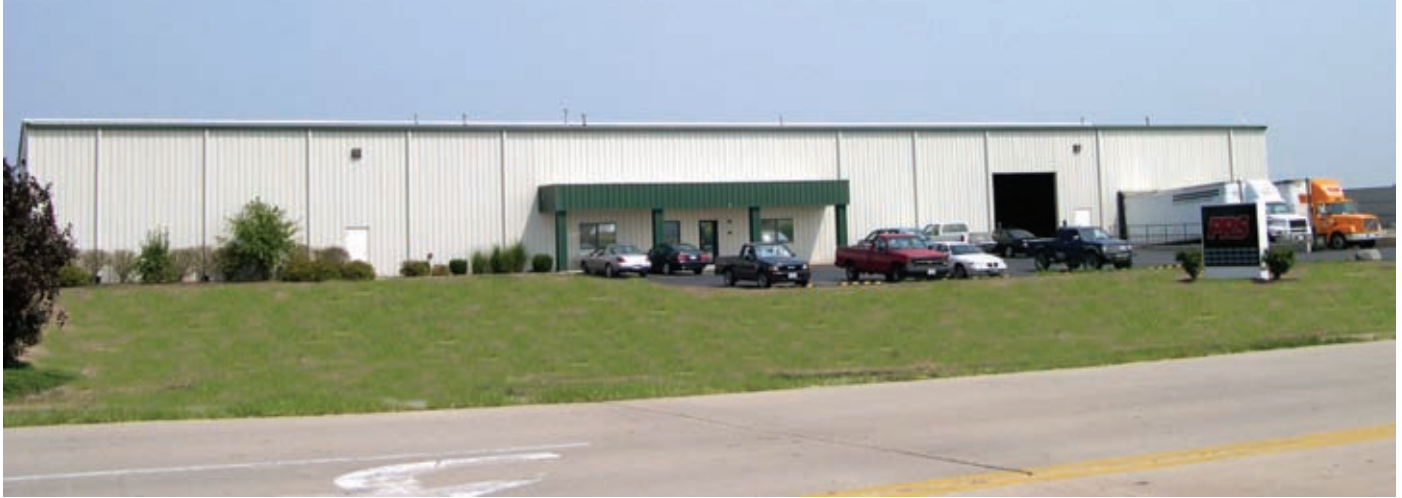
Front view of new 30,000 sq.ft. plant built in 2003. A 12,000 sq.ft. expansion is scheduled.
